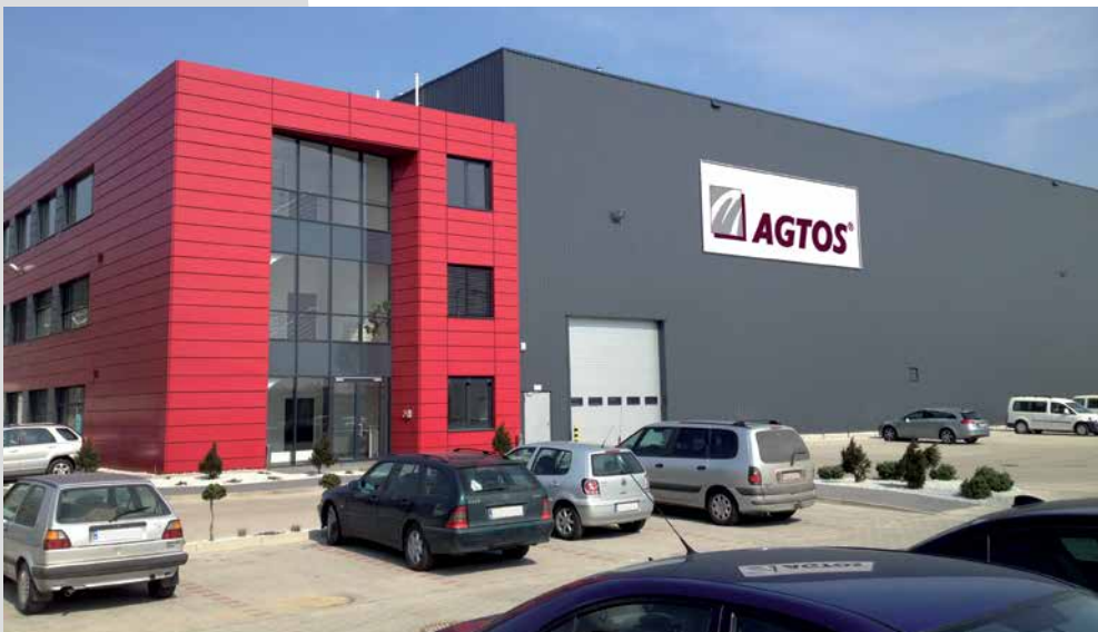
The expanded Agtos plant in Konin features upgraded offices and a doubling in manufacturing floor area.
